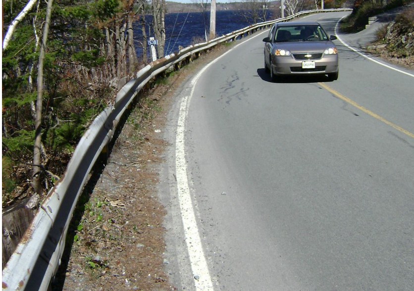
Figure 1. Drivers will often steer across the yellow centerline of the Waverley Road (even on curves) to avoid pedestrians walking along narrow shoulder sections. This maneuver also occurs frequently with respect to clusters of cyclists that use the Road for physical training.
